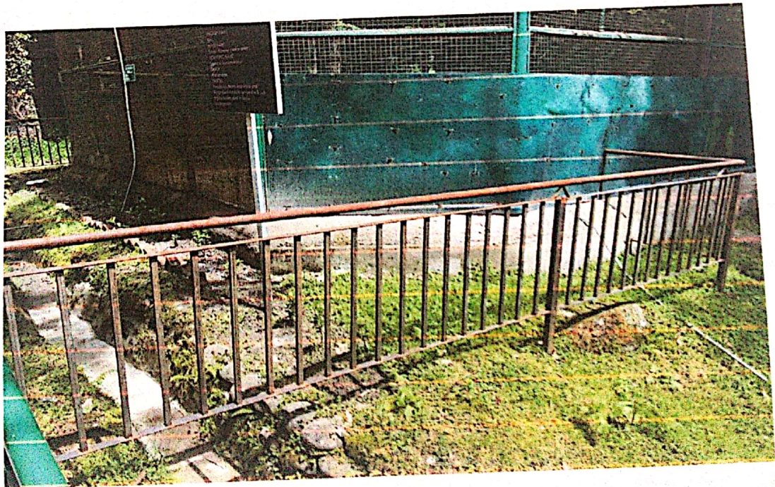
4. Railing / Barrier out side cage .
