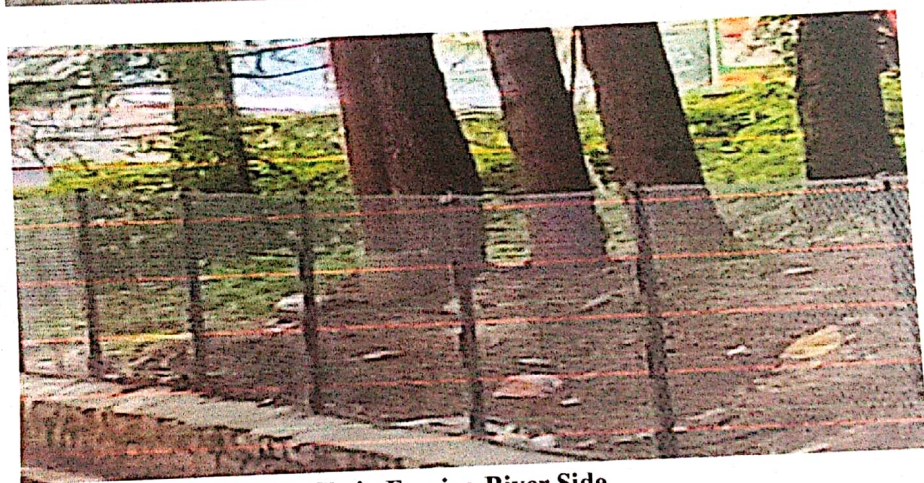
5. Const. of Interlink Chain Fencing River Side
